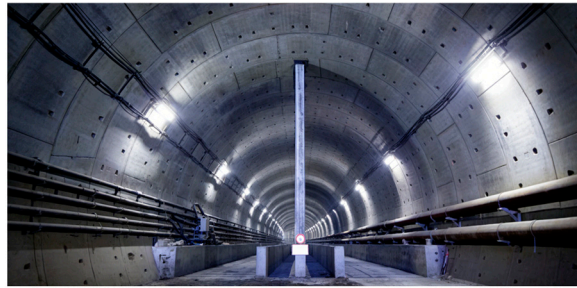
Figure 1: The Groene Hart double-track tunnel with a perforated partition wall.
